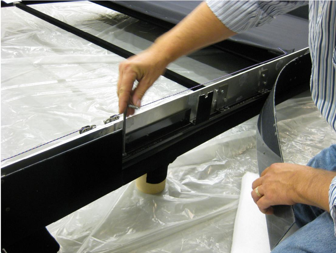
9. Hook up the masks as the picture shows. The (screen) left mask has red tape on it, along with the left mask card, indicating that it is the motor where we reversed the red and black power wires so that it acts opposite of the other mask. The motor power wires are installed into the terminal block either using the included white insertion key, or poking a screwdriver into the upper rectangular slot, depressing the spring that holds the wire.
